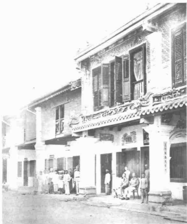
7. The Straits Trading Company offices, c.1900, to which much tin ore was delivered for export, creating a traffic 'black spot'. (Antiques of the Orient)
